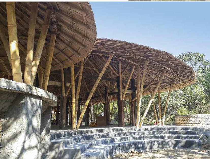
Myanmar: The centre's open and airy multi-purpose hall, which is 25 metres long and about six metres high, is built entirely of bamboo and roofed with bamboo shingles.
