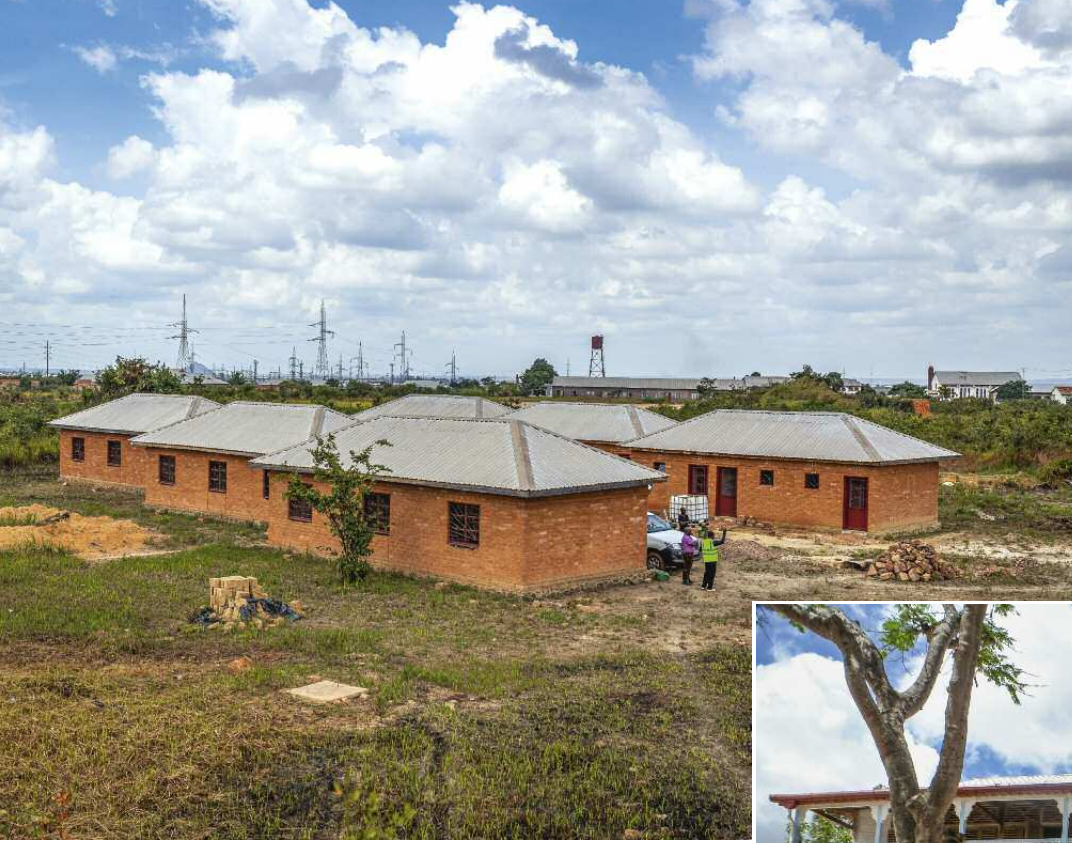
Congo: The training centre is of clay construction (compressed clay bricks). The material was obtained on-site.
