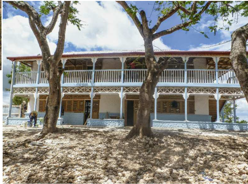
Haiti: The school was built using a mixture of wood and clay (timber frame with clay brick infill). The building is designed to be earthquake-resistant.
