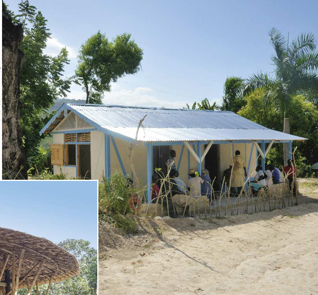
Haiti: This house built on the self-help principle is of earthquake-resistant traditional construction involving timber framing with natural stone infilling.
