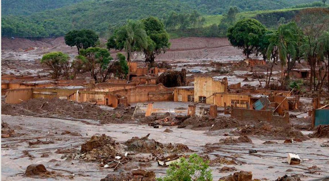
◀ The rupture of the tailings dam of mining company Samarco, owned by Vale and BHP, caused a flood of mud that flooded several houses in the Bento Rodrigues district of Mariana, in the Central Region of Minas Gerais. © Rogério Alves/TV Senado
