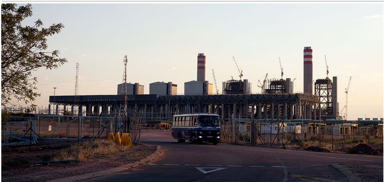
The Medupi coal-fired power plant in Lephalale in the Limpopo region.
