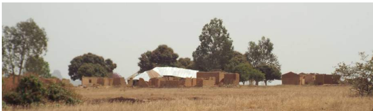
Photo 3. Burnt out houses, Gashish area
