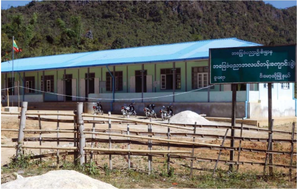
Fig. 16: Middle school in Upper Khupra
