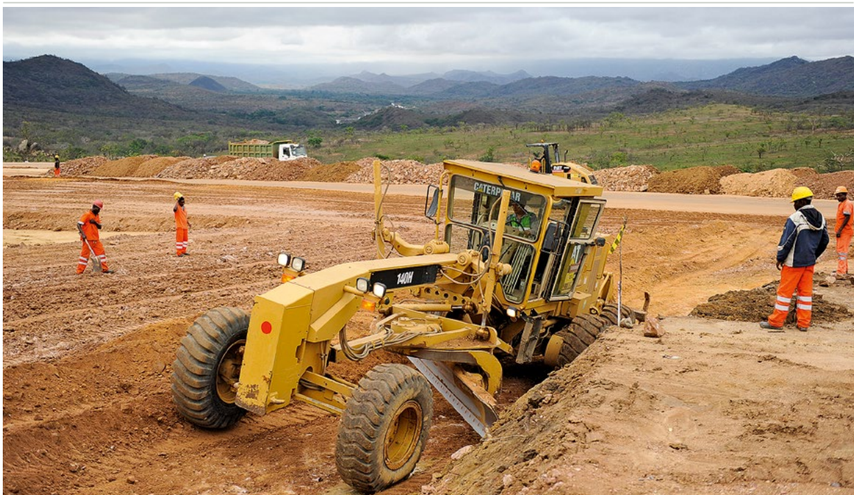
Road construction near Malange, Angola
