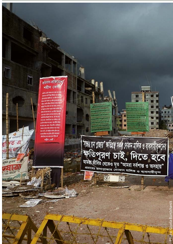
The collapse of the Rana Plaza building in Bangladesh caused over 1100 deaths.
